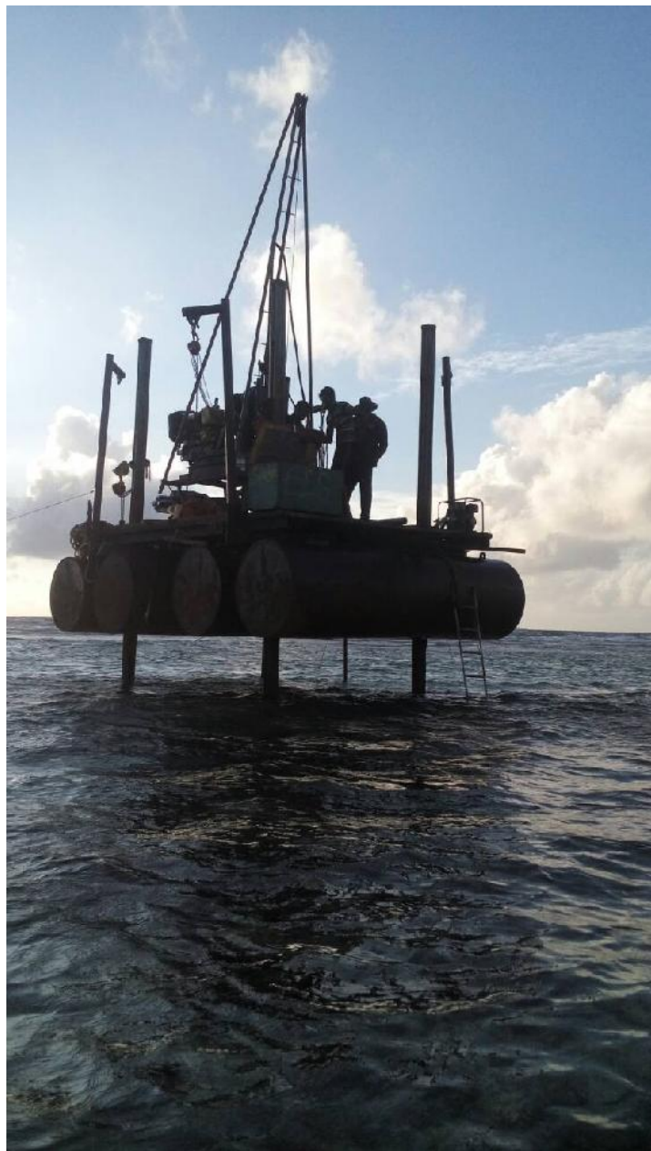
Drilling of Borehole at MBH – 04 location
