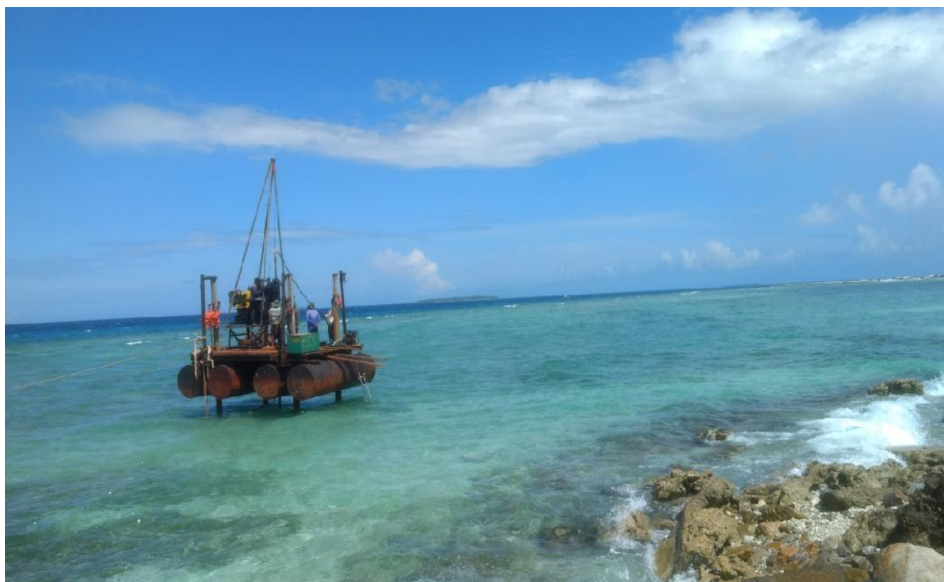
Drilling of Borehole at MBH – 02 location
