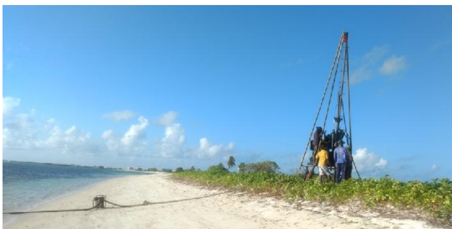
Drilling of Bore hole at LBH-02 location
