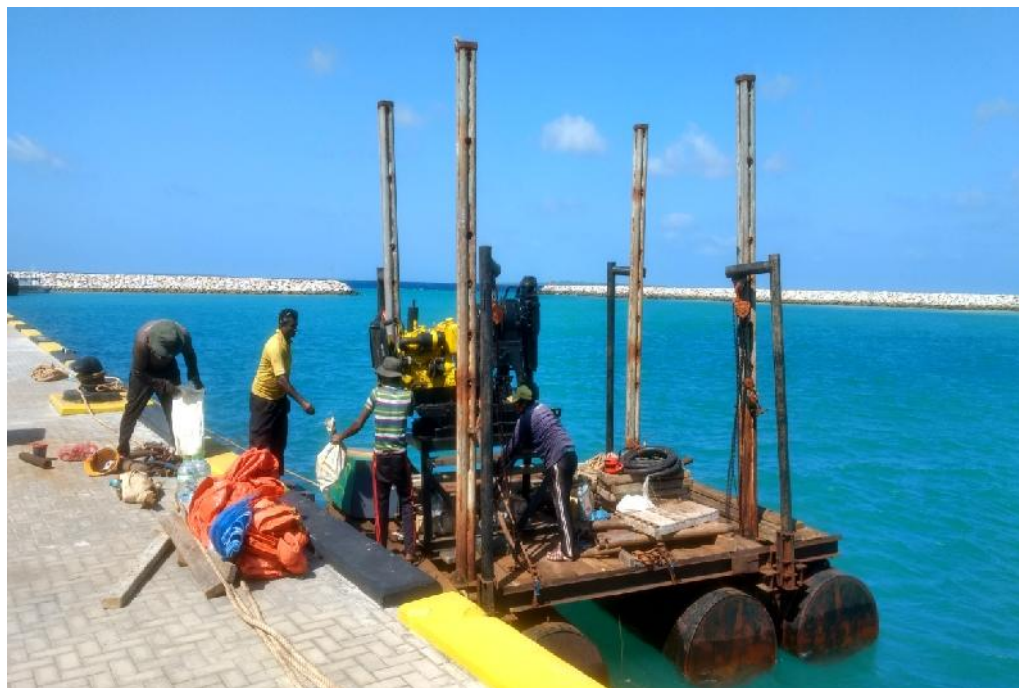
Jack-up Barge Assembling for conducting Marine Boreholes
