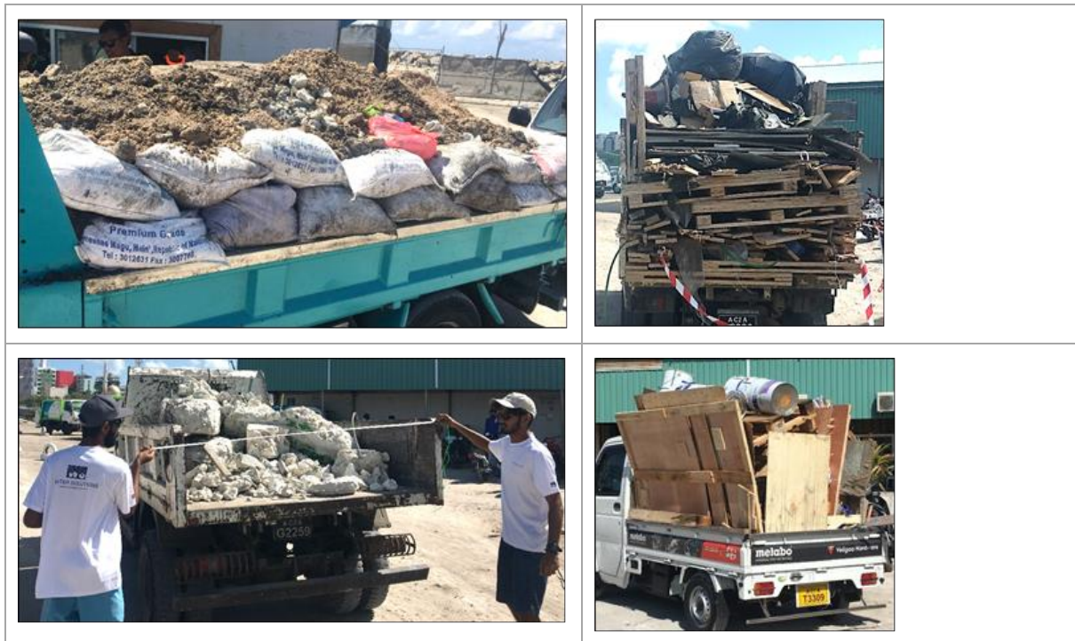
Figure 5: (a) Soil and rock in polypropylene sacks (b) truck overflowing with wooden pellets and other mixed waste (c) Large pieces of demolished concrete (d) Truck overflowing with mostly wooden pellets with some metal containers on top.
