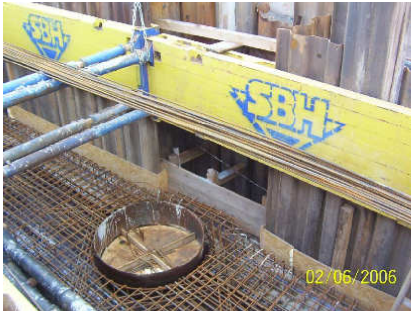
Figure 8 Opening in Reinforcement for Shaft Ring
