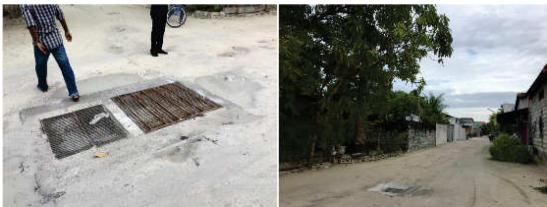
Figure 30: Existing drainage inlets on unpaved roads
