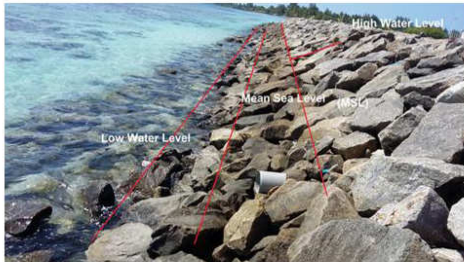
Figure 16 High and low water level at the outfalls
