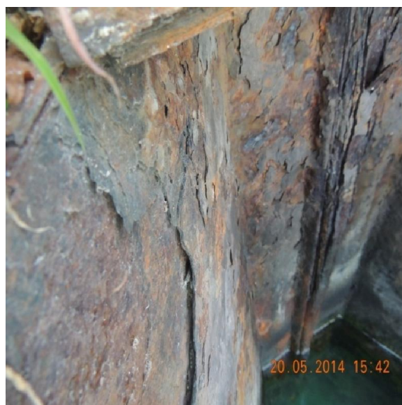
Fig 3.6: corroded steel sheet piles
