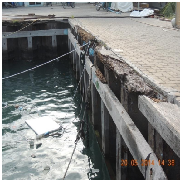
Fig 3.4: Damaged timber fenders
