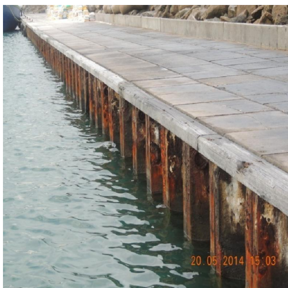
Fig 3.5: corroded steel sheet piles
